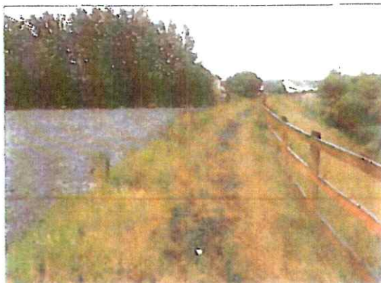
Fig 2. New embankment constructed on eastern site boundary, June 2016
